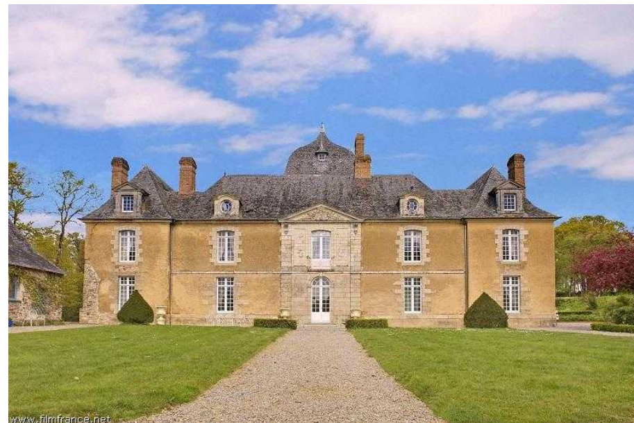
Façade - © ATB / © Berthéléme
