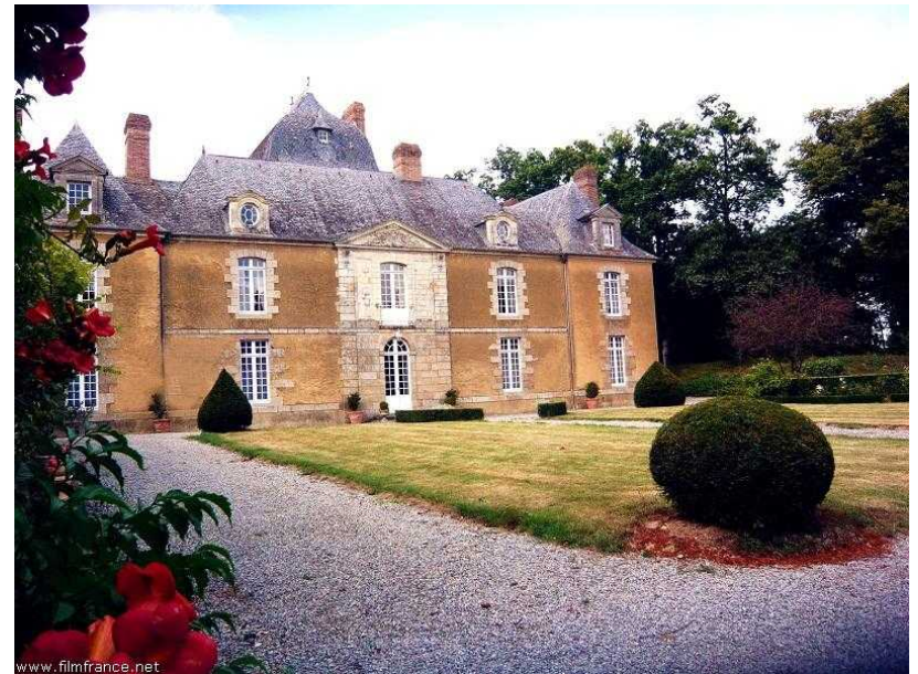
Façade - © ATB / © Berthéléme
